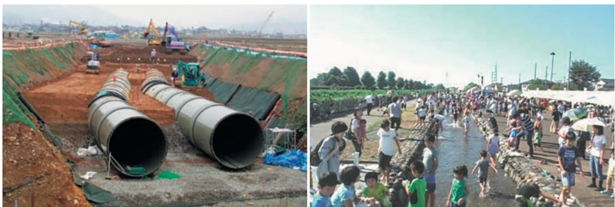
Figure 36: Large scale pipeline and “Seseragi water course” in downstream area of Kuzuryugawa River (Citation: Website of MAFF)
