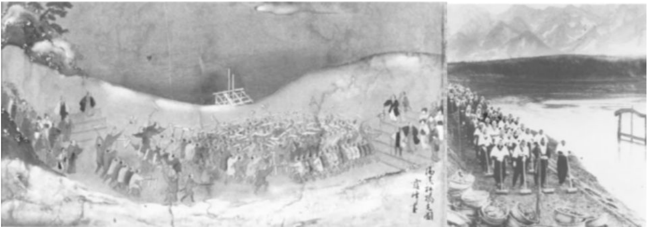
Figure 9: (Left) Manno Ike reservoir - Many laborers compacting the embankment using wooden rammers by the order of a leader
