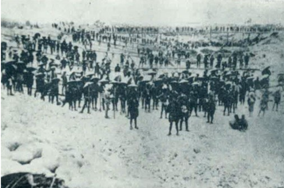
Figure 28: Conditions of Canal Excavation in Jyoganjigawa River (1892) (Supplied by Midori Net Jyousai Yousui)
