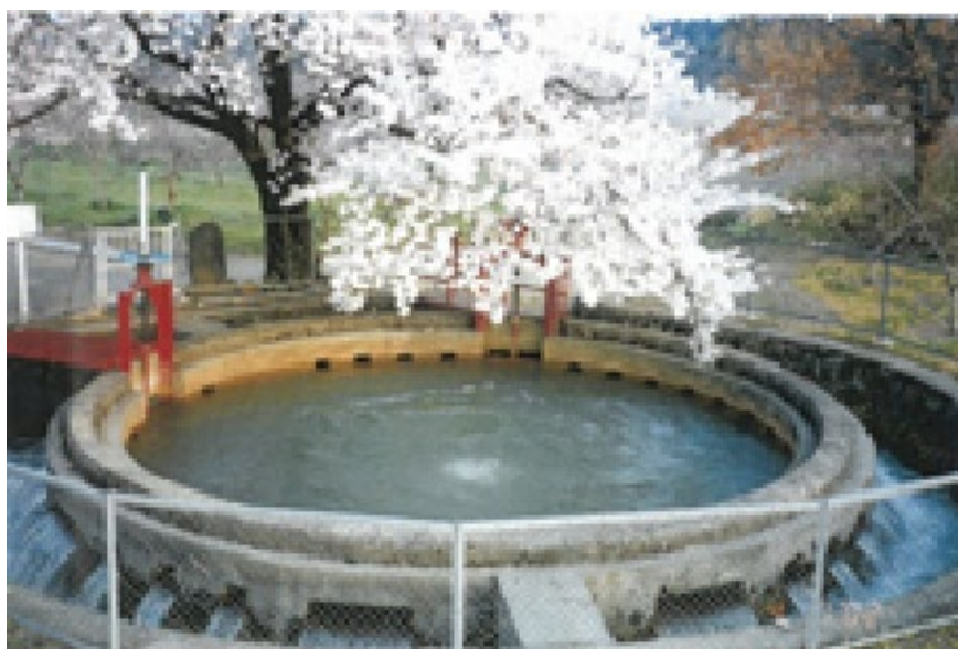
Figure 6: Circular tank diversion works at Kurimoto weir (Fukushima City)
